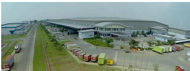
Figure 2: Parking Area to Loading Dock in Distribution Warehouse (Source: mmproperty.com, 2018)
